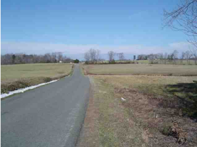
Frontage Taylors Mill Road
